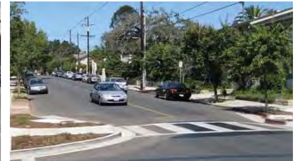
Curb Bulb Out Example
