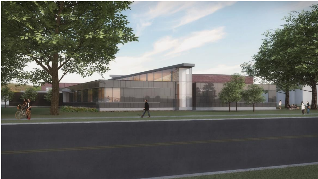
(View from South Broadway)
