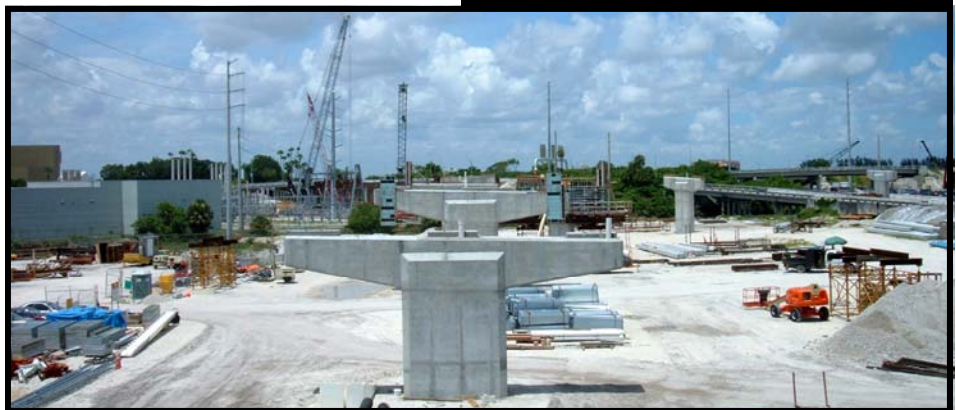
PROFESSORS ADAMS, SCHROER, & DELL VISIT GILBERT- KIEWIT JOB SITE IN FLORIDA
